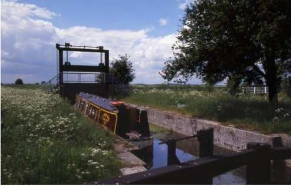
It takes 600 turns of the wheel to raise or lower the gate, so passage up and back would take 2400 rotations.
